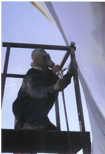
Ecospeed glassflake-based coating is being applied to the chemical tanker Vedrey Barfodh
