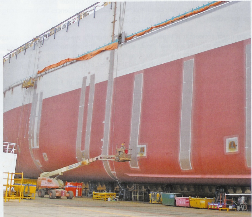
Intergard 787, outside shell at newbuilding.
